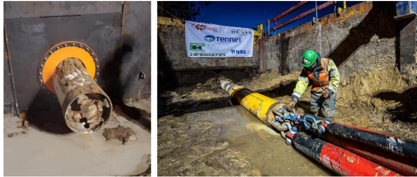
Figure 6. Breakthrough of AVNS machine after pilot drill and pullback of protection pipe bundle of 2,000 m
