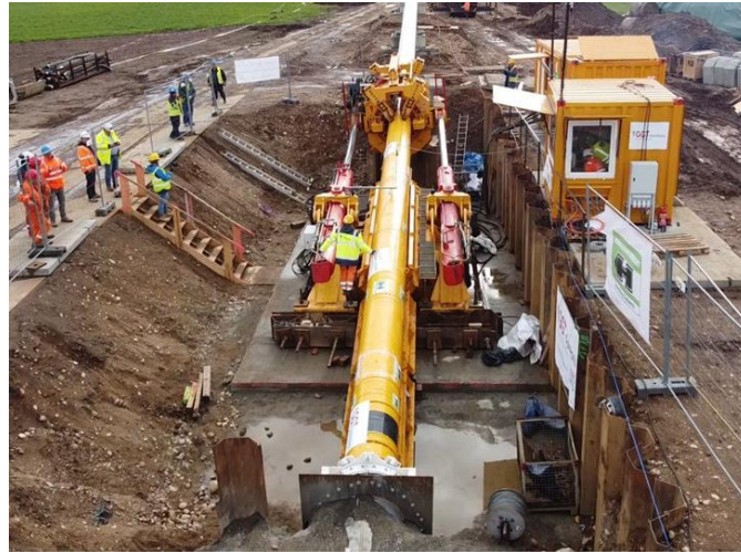
Figure 3. 28" Direct Pipe jobsite installation for 342 m long river crossing in Poland
